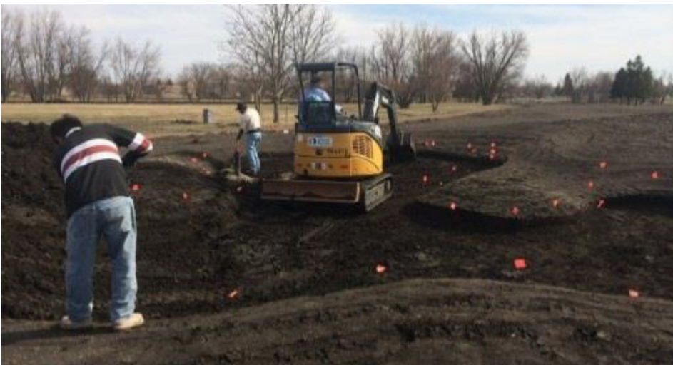
Workers build a new sand bunker to ensure safety of air space 734
